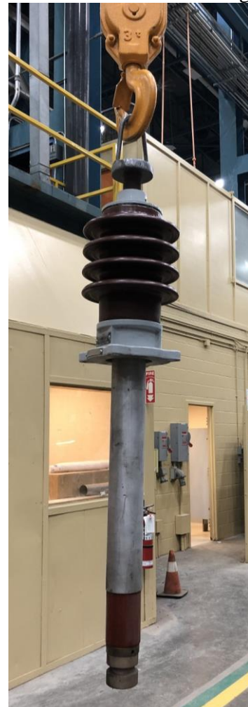
Fig 6 – Lift bushing with lifting eye.
